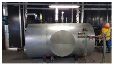
Steam Accumulator, nonfired pressure vessel, correctly sized, ready to supply periodically short bursts of excess steam, supporting the production peak energy demand cycle, the steam generating and distribution system.
