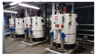
**Boiler steam supply** capacity kg/h and pressure kPa must exceed process demand.
